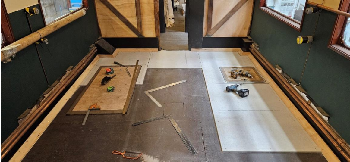
The fire/sound proof layer being laid over the structural floor within the large saloon
