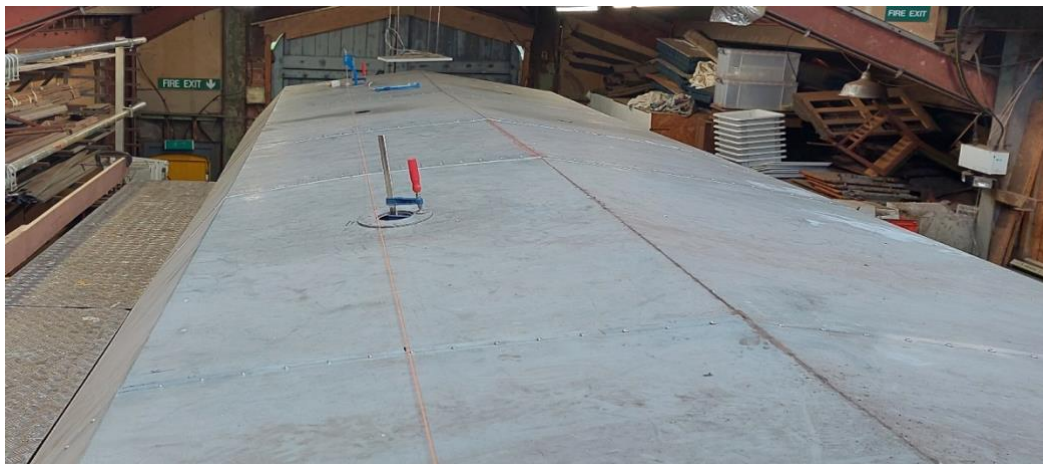
Above: Early roof sheet replacement in progress
