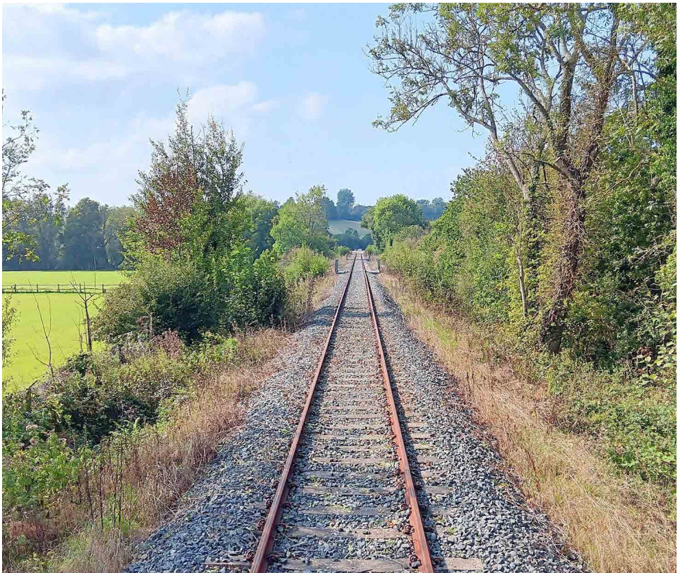
A guard's eye view back from Northbridge Street.
