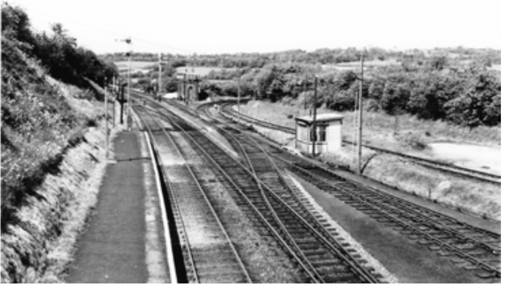
Robertsbridge, looking north, with 'A' box to the right of the picture.
