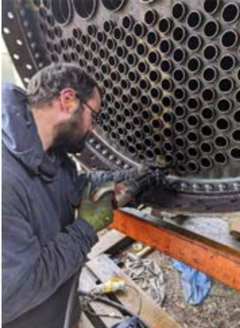
The tubing of 4253's boiler nears completion at HBSS. (via HBSS)
