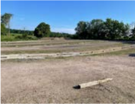
The newly stripped Tenterden car park..
