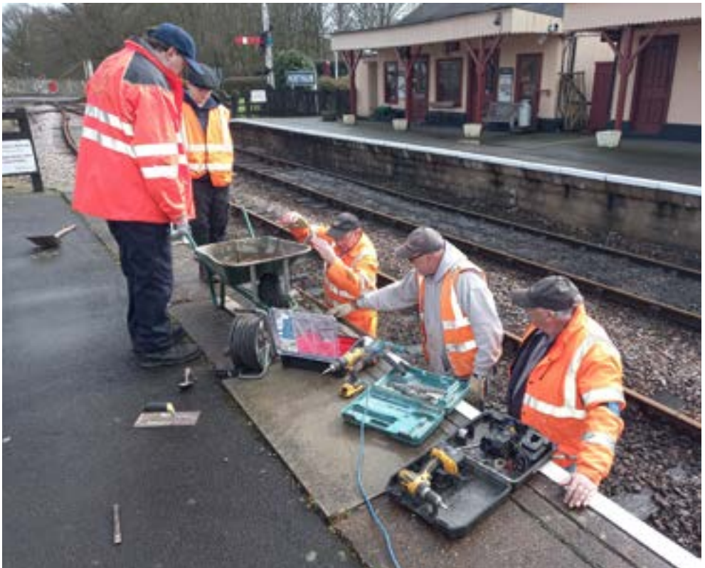
Repairing and repainting the platform edge at Northiam.
