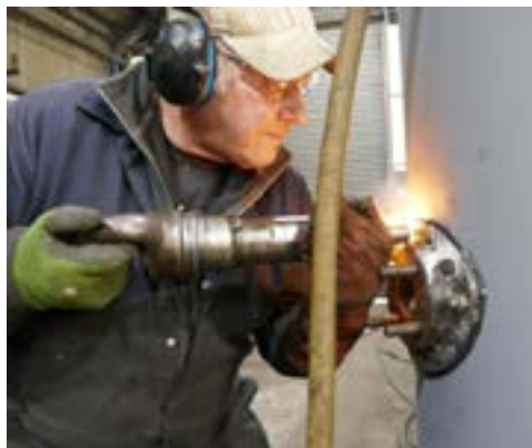
Paul Doel riveting the boss onto 4253's new vacuum reservoir tank. (Charles Masterson)
