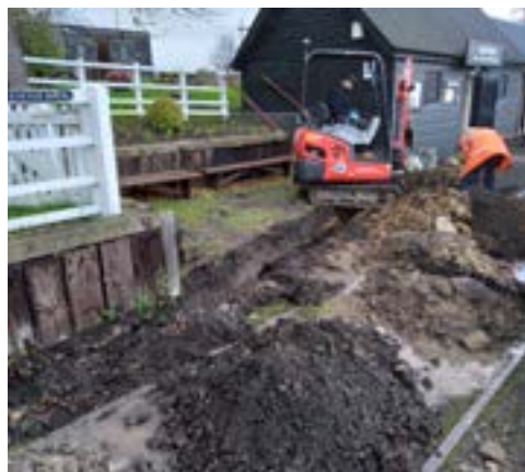
Digging the cable trench. (Malcolm Burgess)
