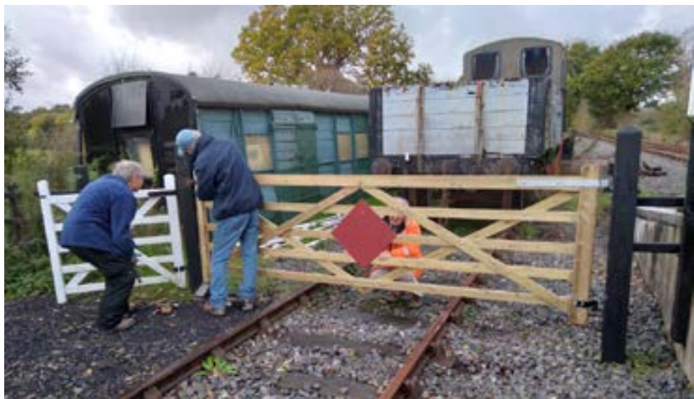
The new rail gate being fitted.
