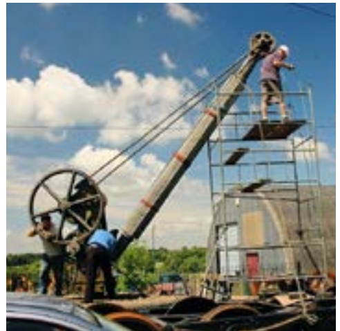
The yard crane under repair at Tenterden.
