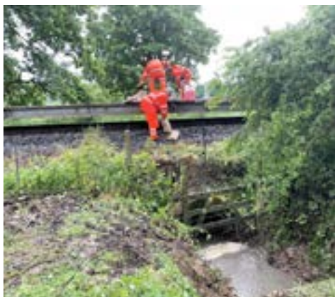
Clearing the culvert. (Paul Jessett)
