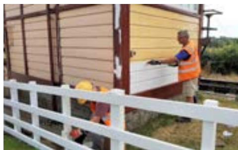
Fresh paint being applied at Wittersham Road.
