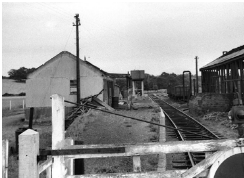
The site being cleared by British Railways in July 1955.
