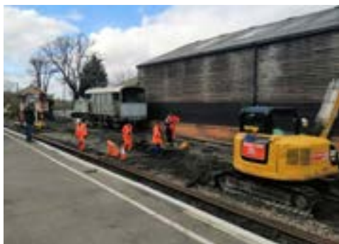
The Tenterden loop relay in progress.
