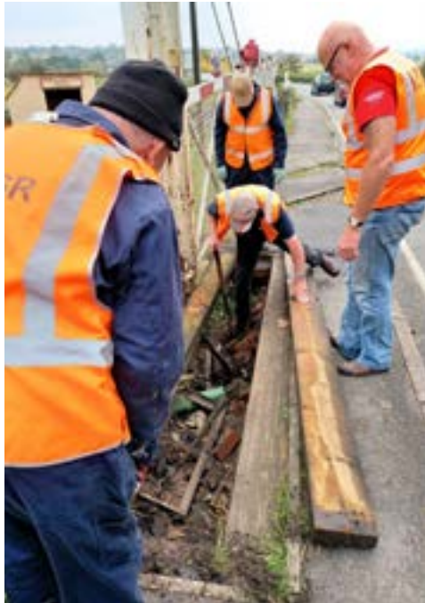
Replacing rotten timbers at Northiam crossing. (Graham Hopker)
