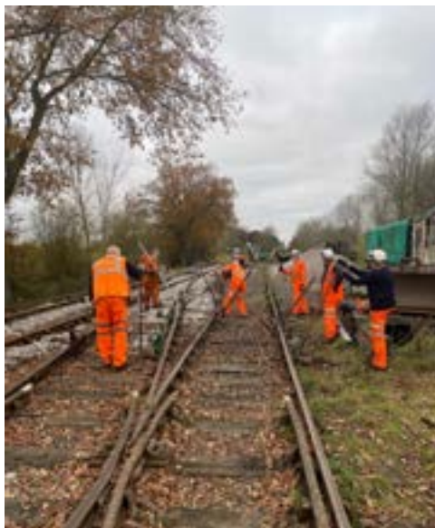
Members of the P.Way Department levelling up the spur road. (Paul Jessett)
