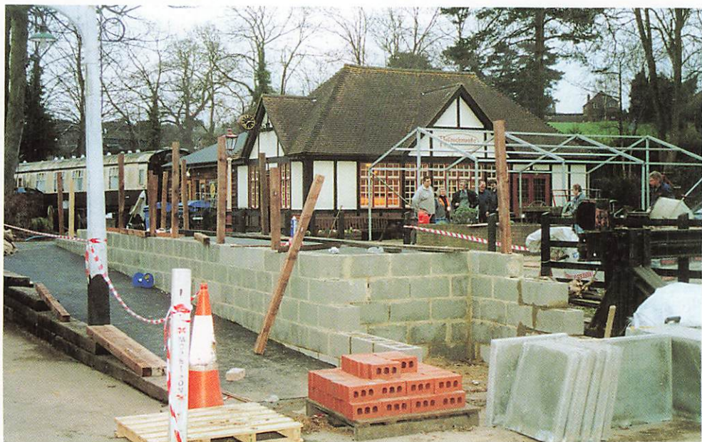
The new disabled access ramp to the Pullman dock under construction by the Tuesday Group, 5 February 2005.
