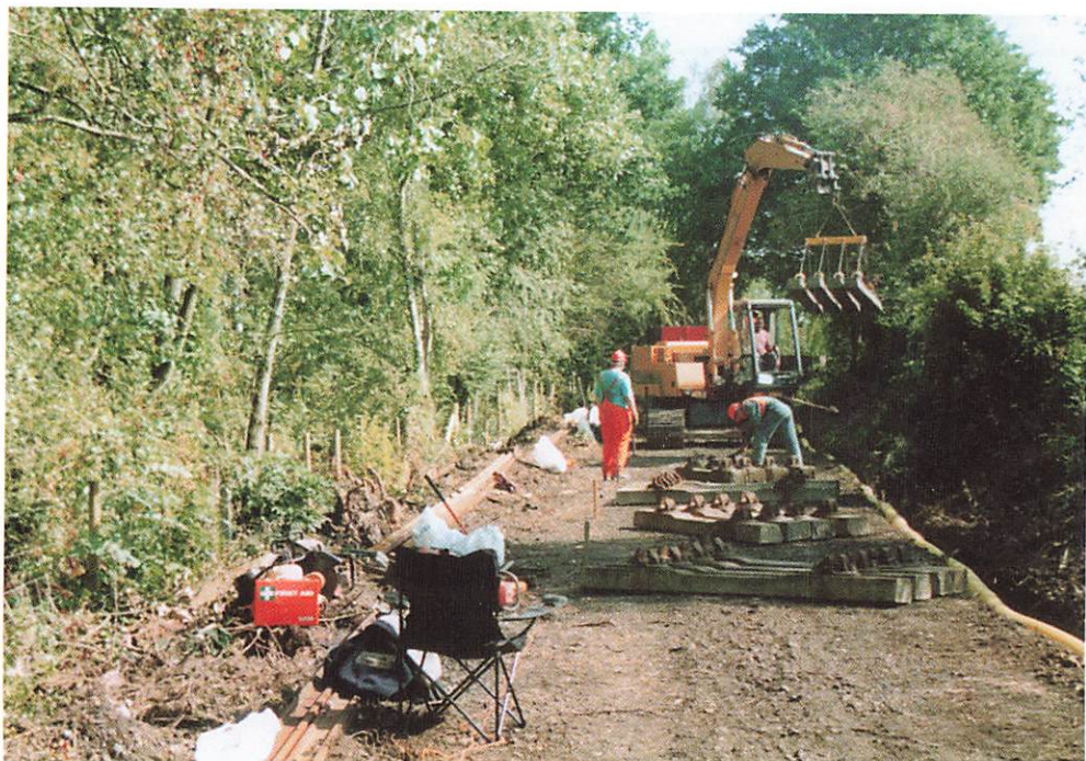
Track laying in progress in the long siding beyond Bodiam, 2nd September 2004
