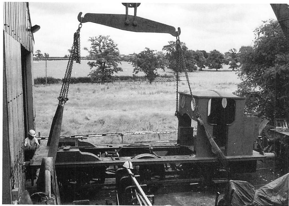
36 ton crane lifting No 3's frames on to the motion outside Rolvenden Shed, on its return from Ian Riley, Bury. (Tom White)
