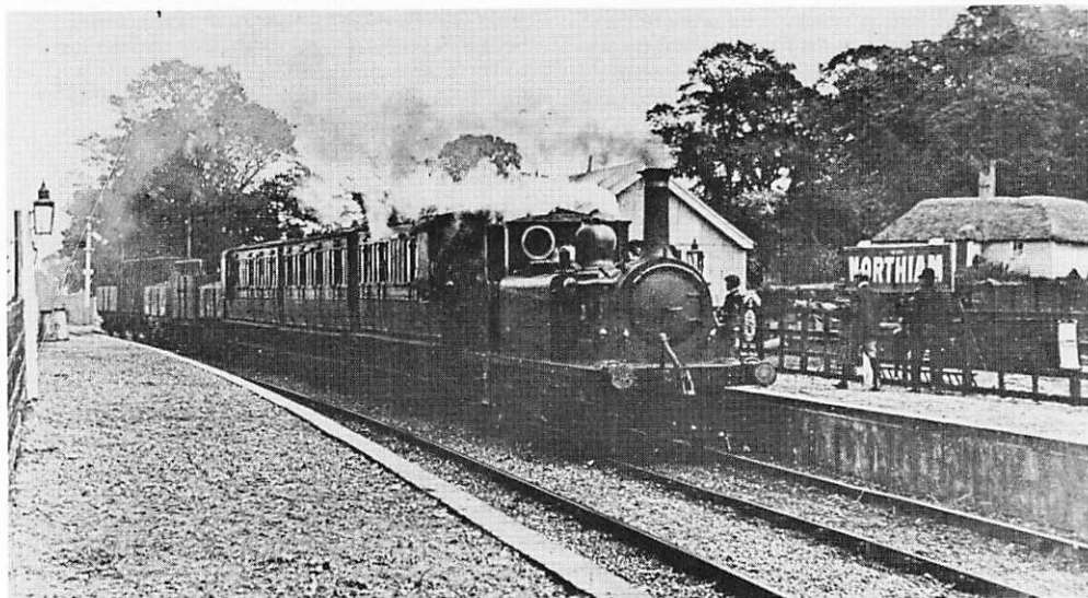
Northiam Station, circa 1901. The locomotive is No. 3 "Bodiam", still with condensing pipes as delivered. These were removed in 1904
