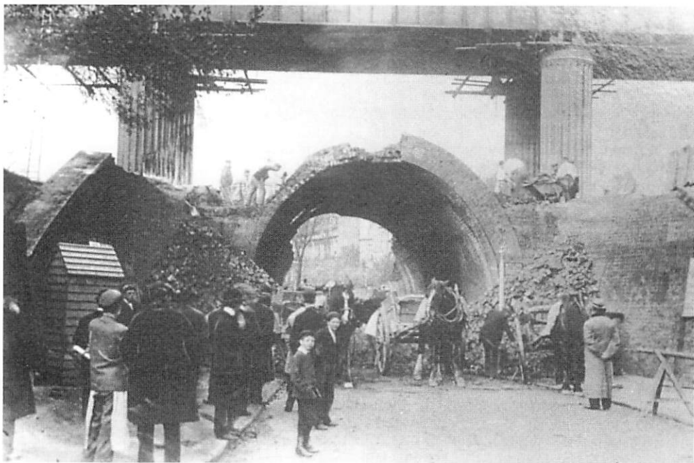
Queens Road, Hastings, in 1898. The new road bridge is complete and the old embankment is being dug out and carted away. (David Padgham collection)
