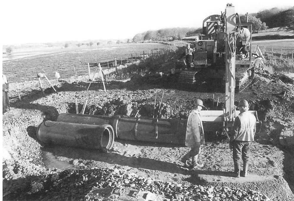
Laying in new balance pipes at Mill Ditch to counter the flooding problems seen last year, 21st November 2001, the cost of these works was around £20,000.
