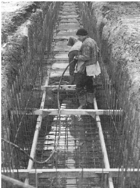
The floor of the new C&W inspection pit at Tenterden under construction (Peter Salmon)
