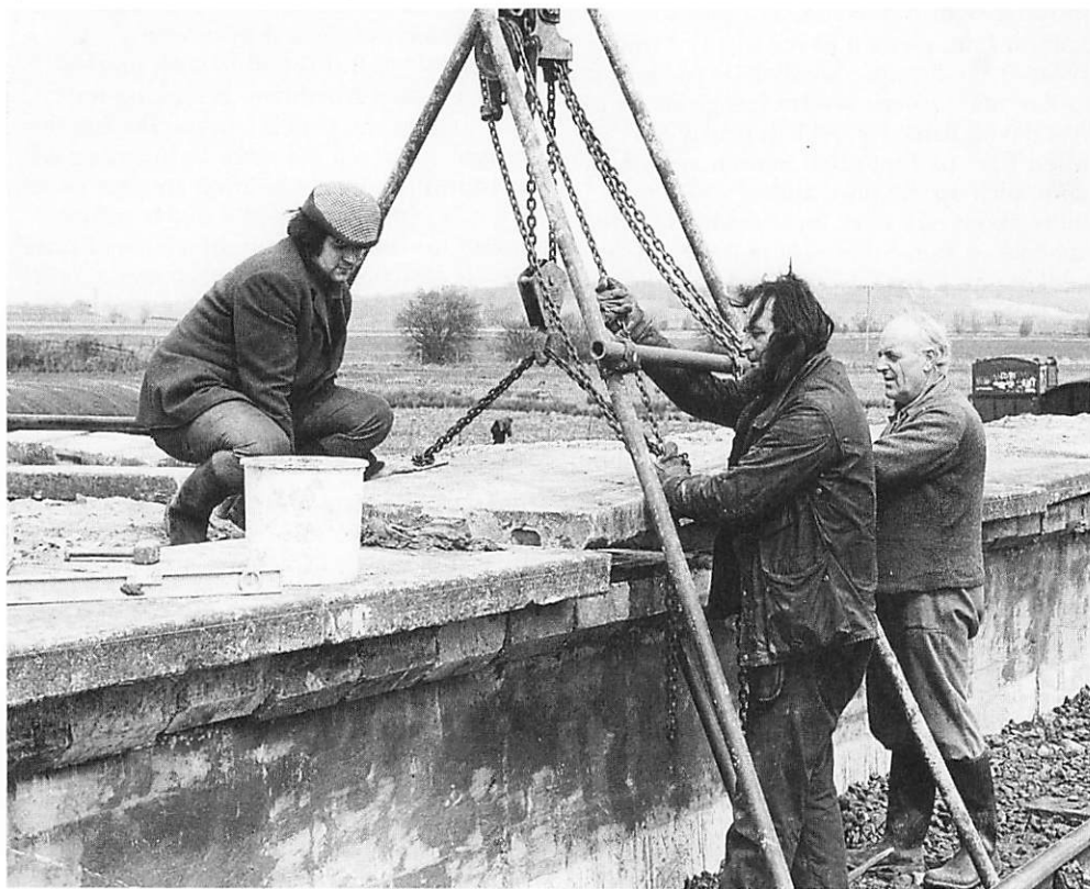
Lifting the Heathfield coping stones into position at Wittersham Road (L-R) ?, Dave Harris, Dave Levett
