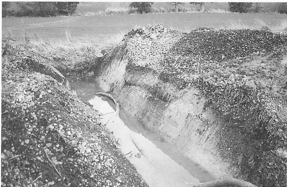
Cross section of track as cut away for a new cross drain at Willow Curve.
