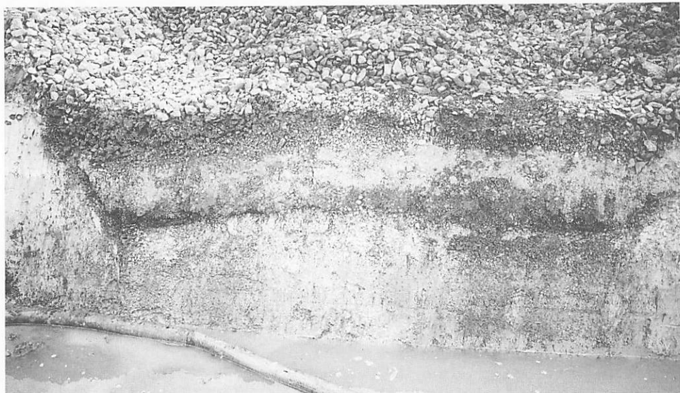
Close up of cut away section of embankment, showing (from top) stone ballast, permeable layer, ash ballast and impermeable clay. (John Liddell)
