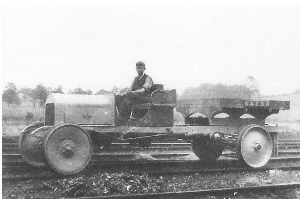
The chassis of the Wolseley Siddeley railbus at Rolvenden, probably 1921
