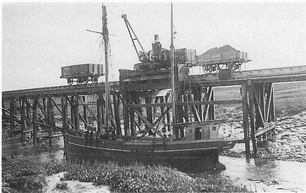
The 'Lily' at Wick Wharf, probably 1927. Note steam crane which appears to have completed unloading coal into the private owner wagon (centre) and WC & PR wagons 25 and 11 (left and right).
