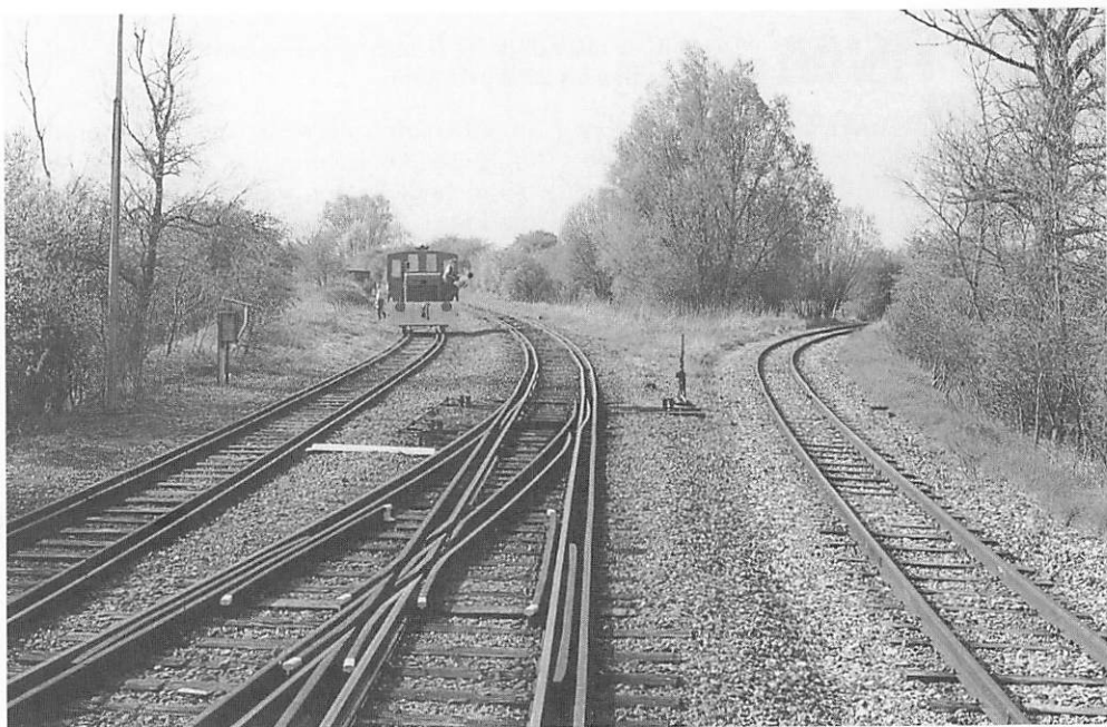
Dual Gauge trackwork outside Noyelles. The line to Le Crotoy is on the right, 27th April 1996.
