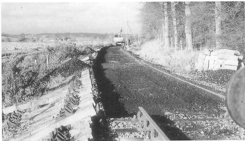
The old wooden sleepers removed and track bed dug out ready for concrete sleepers (ready on left): 12th January 1996.
