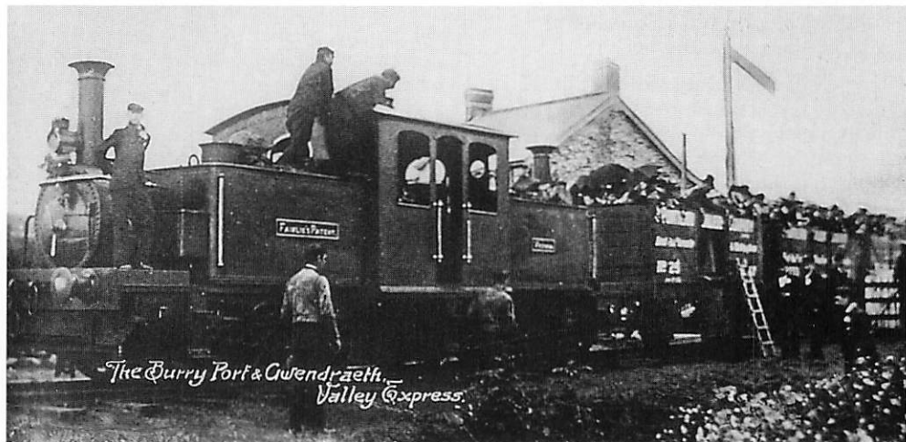
'Victoria', a Fairlie Patent 0-6-6-0T, built in 1866 and rebuilt to standard gauge in 1873 on a miners' excursion train of Pontyberem Colliery Co. wagons in the late 1890's.
