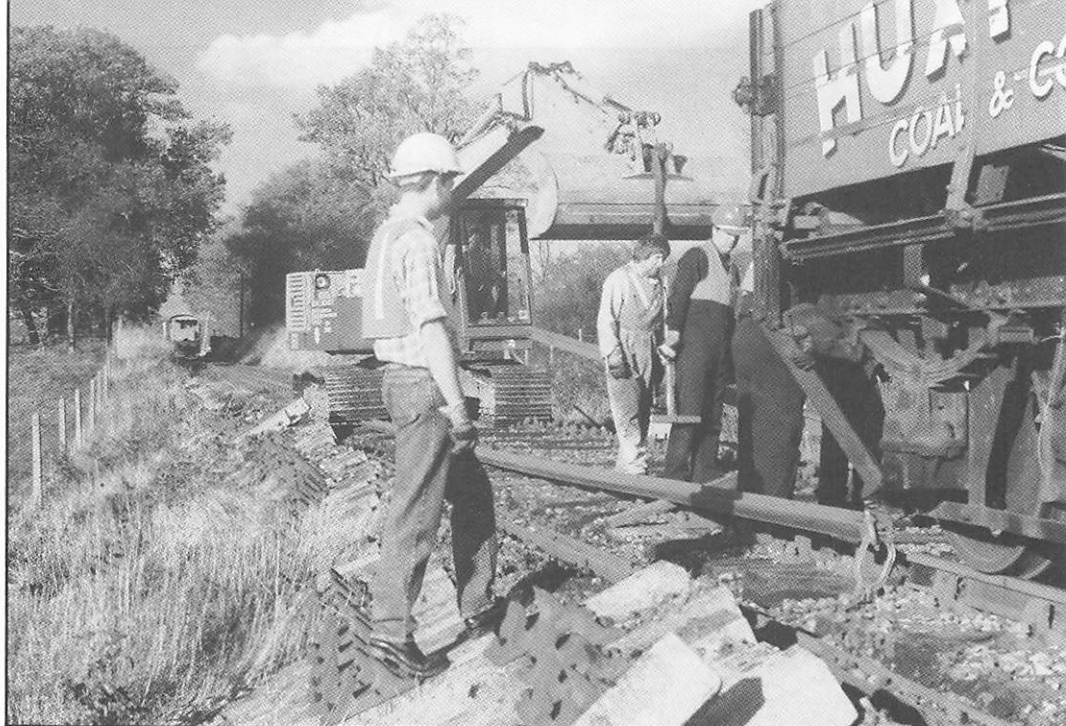
The P. Way gang ripping out the old 91 ¼lb rail at Gazedown Wood, 7th November 1994. (John Liddell)
