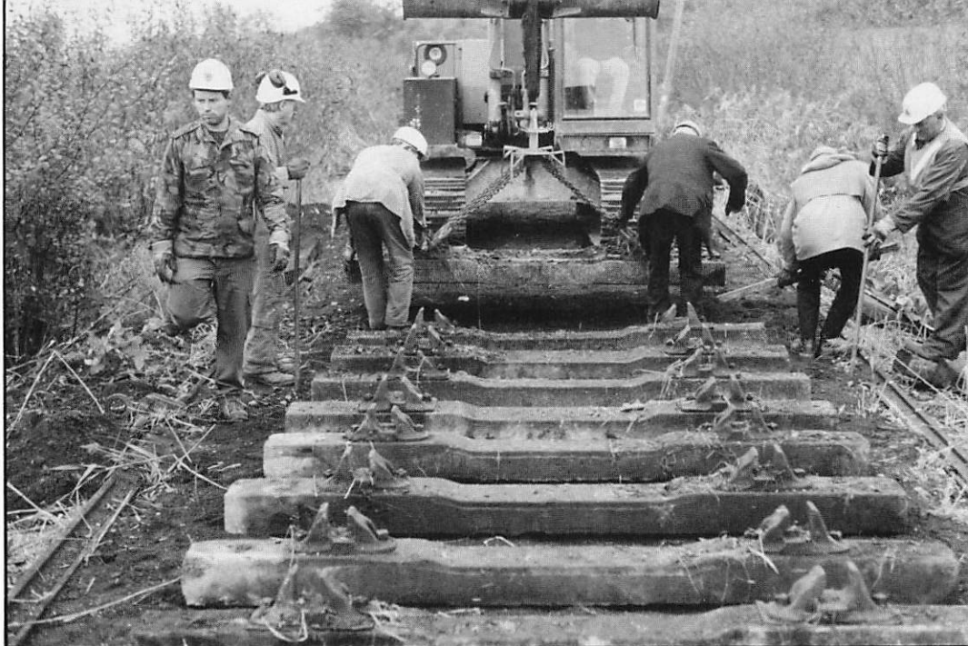
Track relaying between Newmill Bridge and Gazedown Wood during November 1993. Concrete sleepers are being used to replace the existing worn out wooden ones. (John Liddell)
