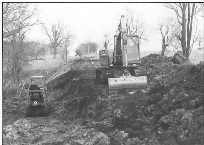
Embankment removal using contractors' plant.
