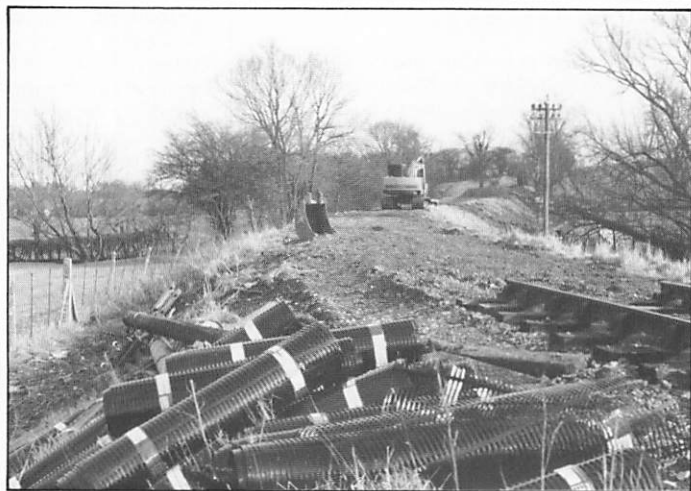
Specialist netting to stabilise the new embankment.
