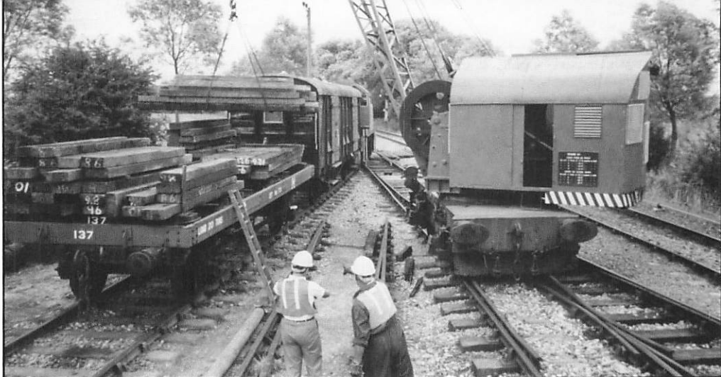
Unloading point timbers in the permanent way sidings at Wittersham Road in preparation for replacement in the point adjacent to the signal box, 11th July 1992. (John Miller)
