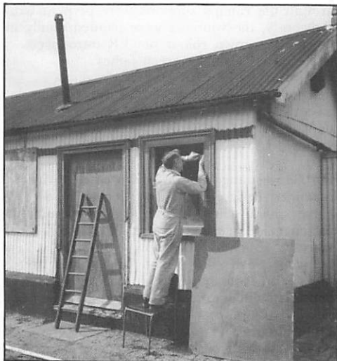
Bodiam, 26th April 1992. Ken Lee removes the sash window from the Parcels Office for refurbishment, and infills the corrugated iron roofing to prevent rainwater entering.
