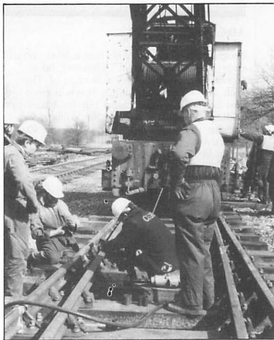
Installing the new point at the Rolvenden end of Wittersham Road. (Maureen Moore)
