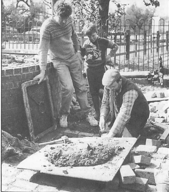
Laying granite setts outside the carriage shed.
