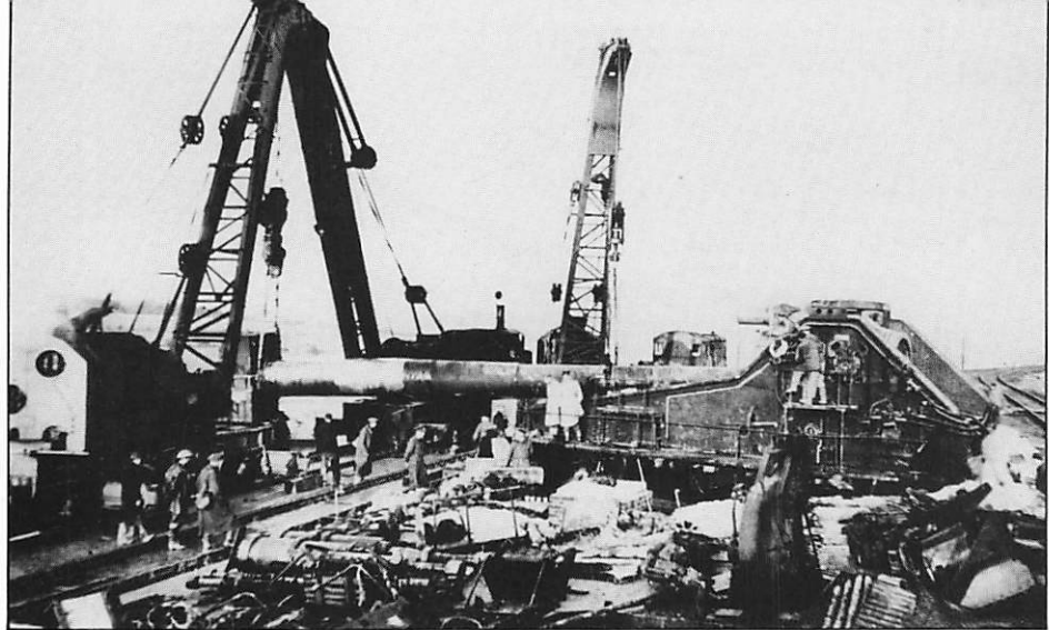
Three railway cranes change "Pooh's" barrel, St. Margaret's-at-Cliffe, 1940. Note rail loops provided for the purpose. (D. G. Collyer collection)
