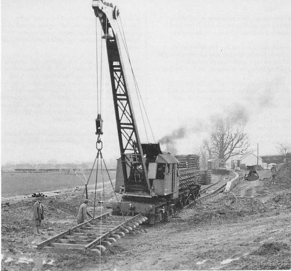
Laying temporary track panels at Northiam to accommodate spoil trains, Boxing Day 1989. (Brian Stephenson)
