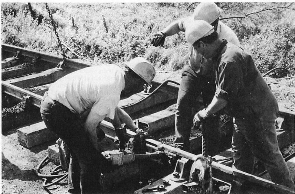
Gary Barker and the railhead team bolting up fishplates on 15 May 1989.
