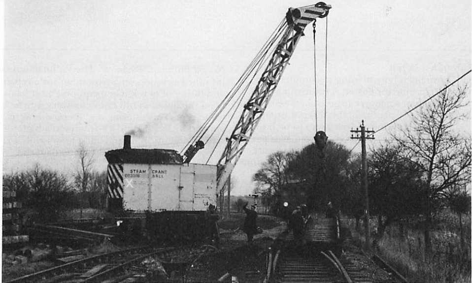
P.W. department staff laying in new pointwork at Wittersham Road with the aid of the Grafton steam crane, No. 145, on 15 January 1989. (Neil Rose)
