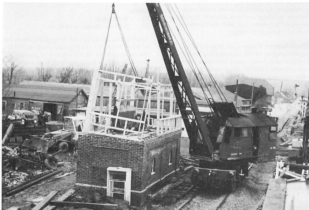
Erecting the timber framework for Rolvenden Signal Box on 12th April 1988 (David Stubbs)
