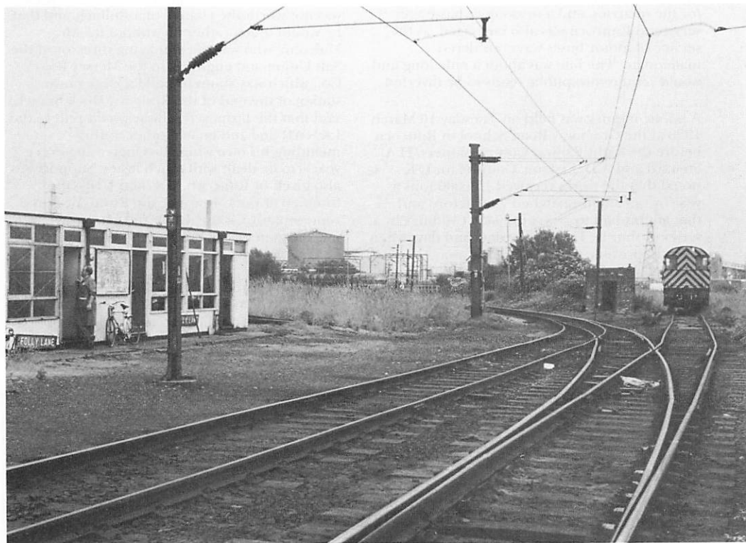
The start of the Weston Point Light Railway at Folly Lane. The WPLR branches to the left, the line continued straight on to the MSCC Railway and the siding to the Mersey Power Company. Percival Lane Power Station diverged to the right (Philip Shaw)
