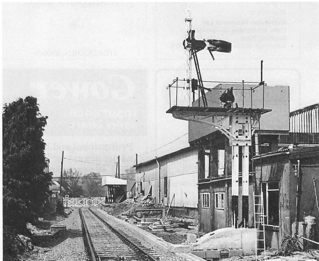
Newly restored track formation at Rolvenden, awaiting re-instatement of the platform, 7th May 1988 (Brian Stephenson)
