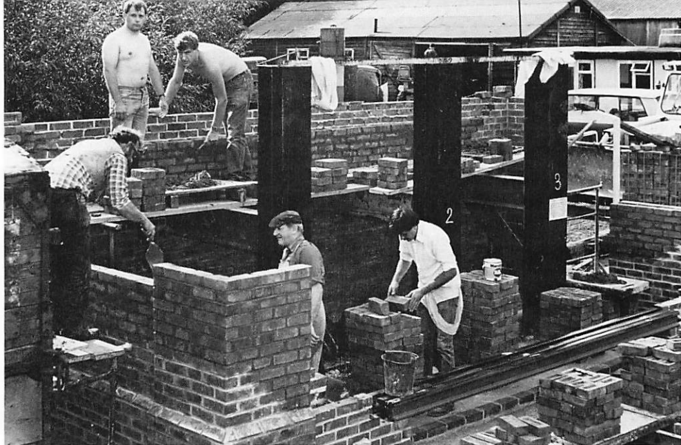
The signal box at Rolvenden takes shape. Compare with the picture of the foundations, somewhat inappropriately included in the Wadhurst Rescue article on page 35 of the summer issue. (Brian Stephenson)
