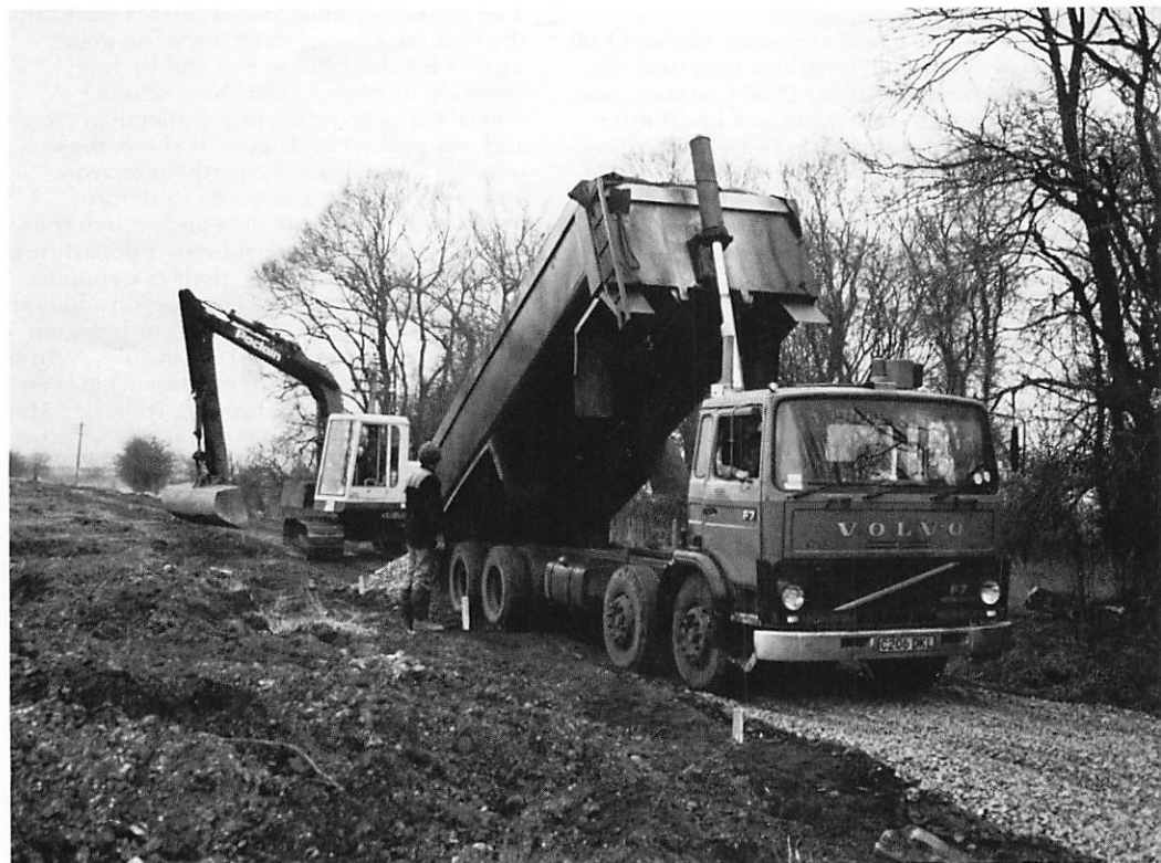
David Hazeldine watches carefully as a load of Irish minestone ballast is emptied on to the track bed on the operating section near Wittersham Road, March 1987 (Paul Sutton)
