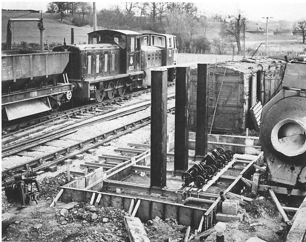
Foundations in place to take the re-erected signal box at Rolvenden, 18th April 1987
