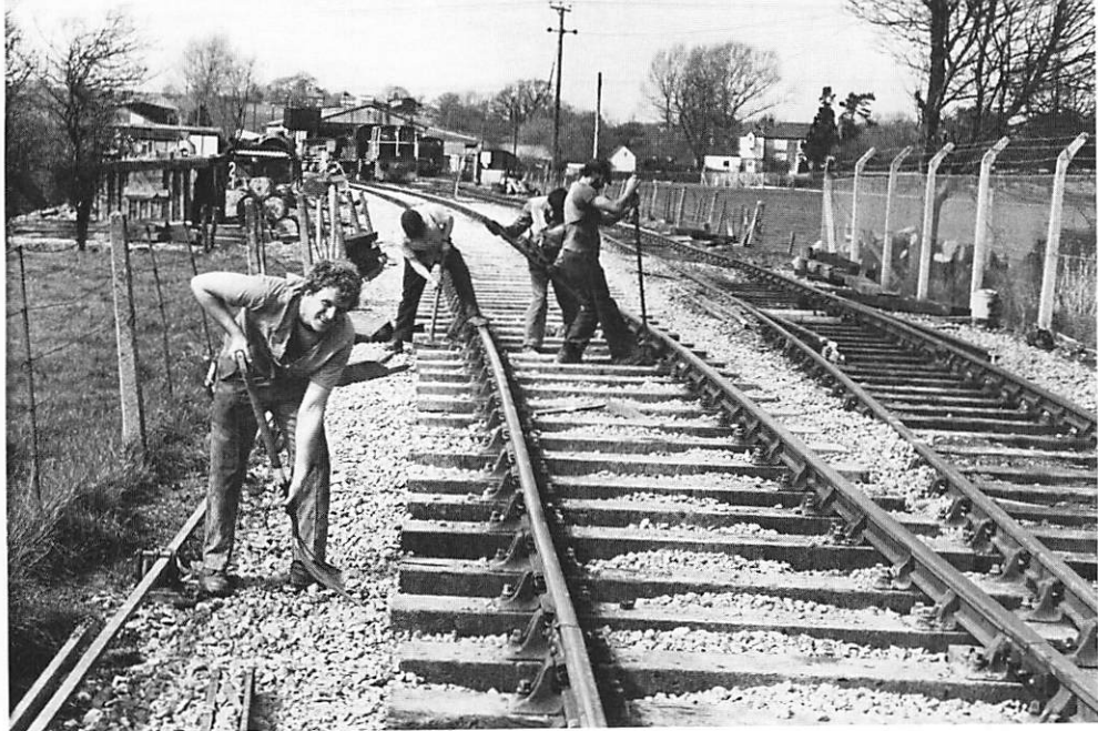
The permanent way gang at work jacking and packing the track outside Rolvenden on 18th April 1987. The author is on the left (Brian Stephenson)
