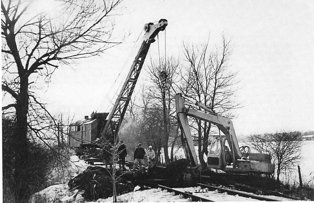
Replacing the dry culvert with plain track, near the Oxney Straight, 11 January 1987. [Brian Stephenson]
