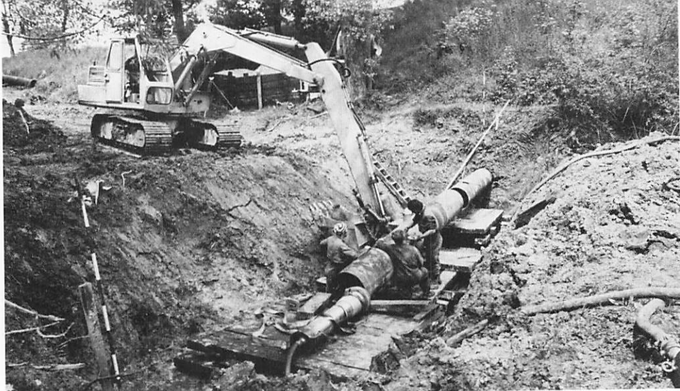
The Hymac aligning another section of pipe in readiness for welding to that already part buried in the bank. The Jack Hammer lies waiting ready for action. June 1986 [Robin White]
