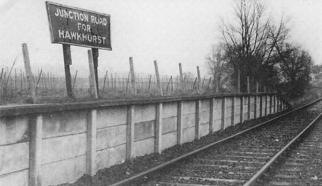
The "new" Junction Road with standard S.R. type concrete platform units and fence posts to match.
