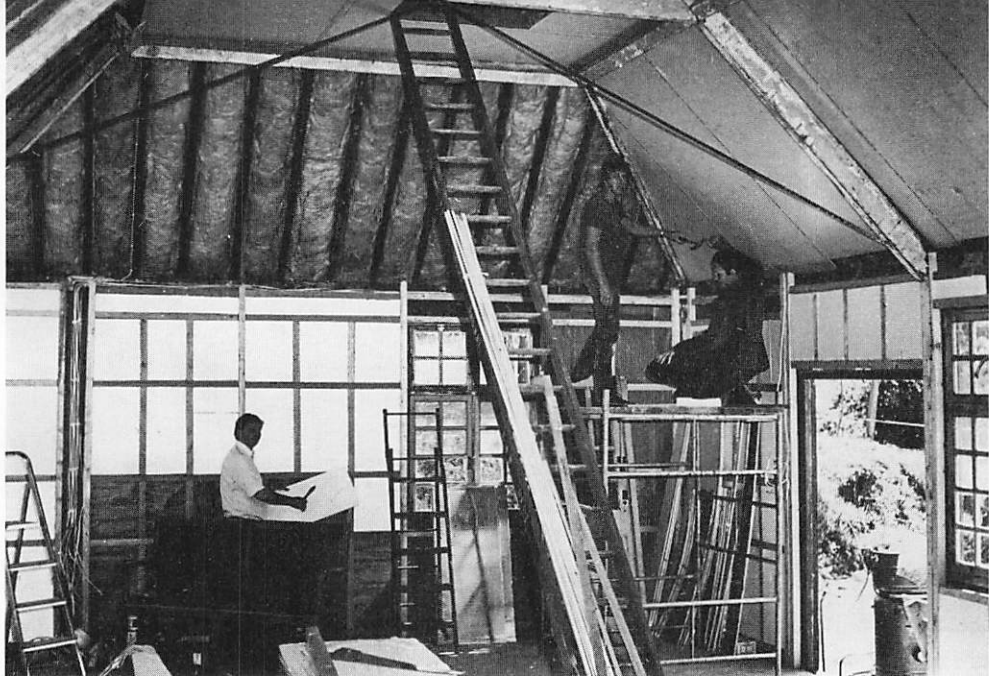
The inside exposed! Tacking up plasterboard in the new catering building. L to R: John Miller, Dave Stubbs and Allan Tebboth, 25th May 1986 [Brian Stephenson]
