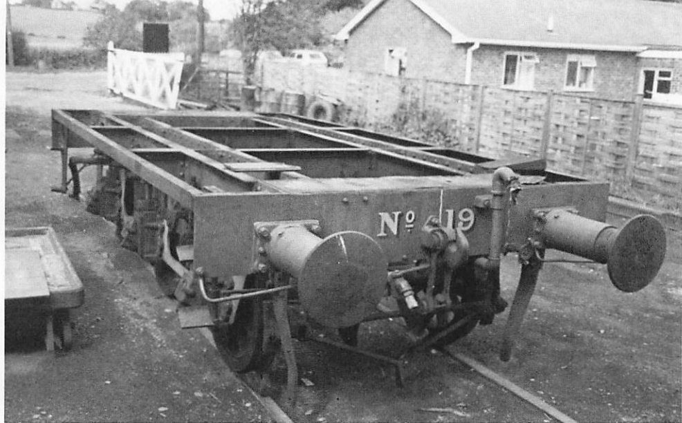
The chassis from No. 19's tender parked outside the west end of the shed at Rolvenden, 15th September 1985.
