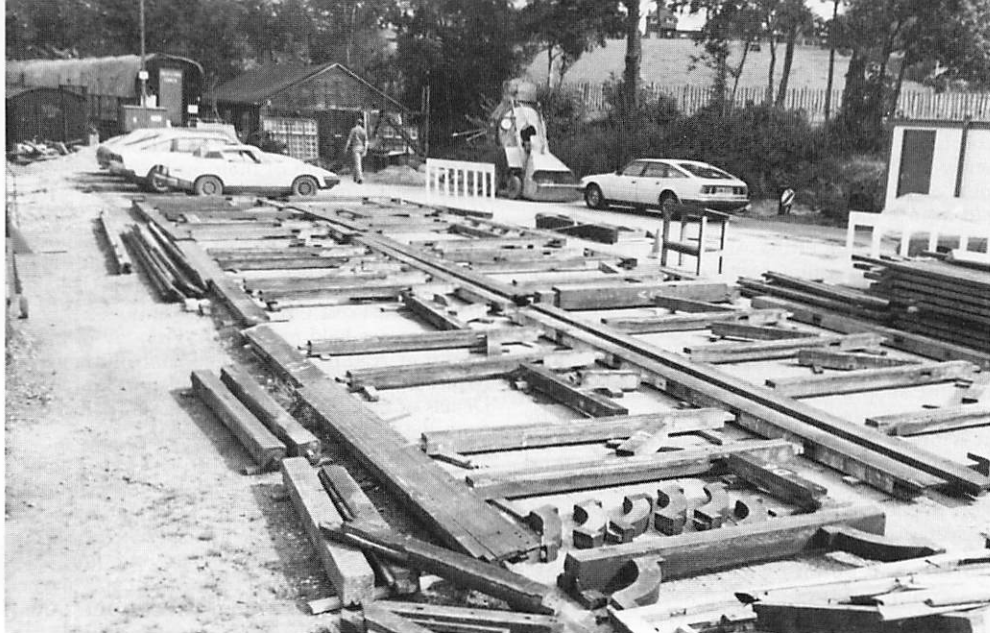
Bus station office laid out prior to erection in Tenterden Yard, 15th September 1985 [Paul Sutton]
