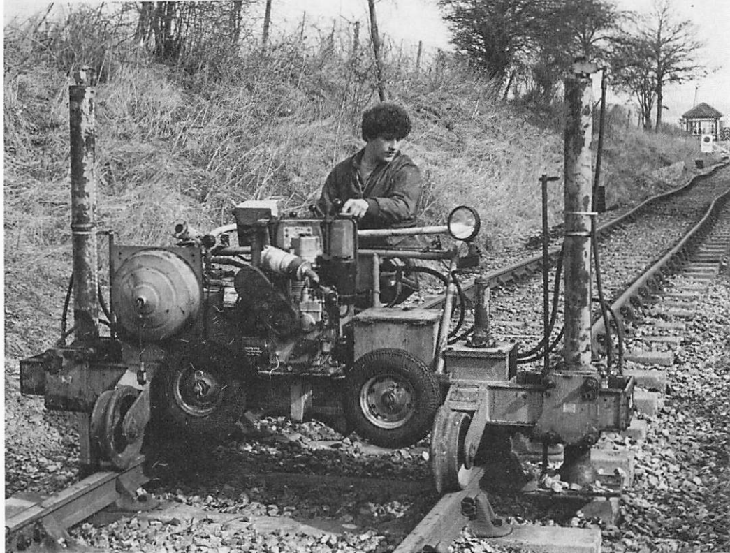
Franz-Plasser track lifting and slewing machine in action on Wittersham Bank, operated by B.R. employee Mark Margerison, 23rd March 1985 [Hugh Nightingale]
