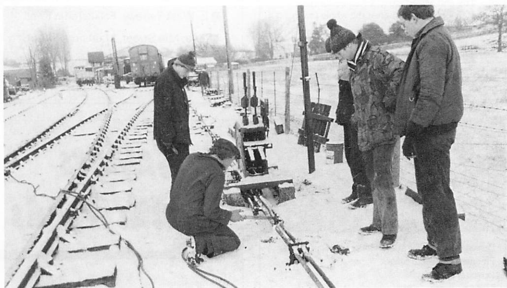
Dave Hazeldine burns off seized up bolts on point rodding, watched by members of the Signal & Telegraph department, 6th January 1985
