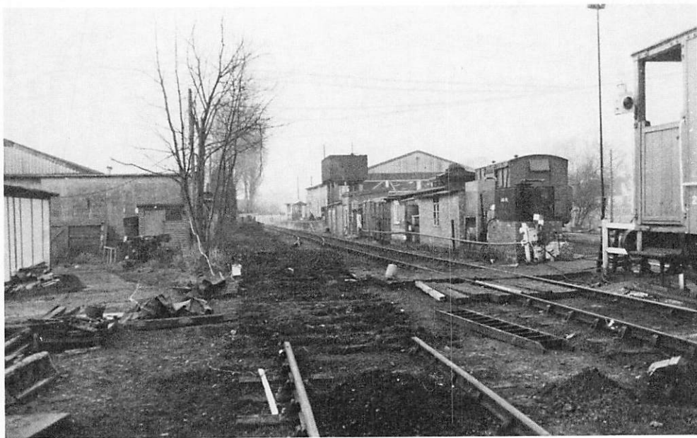
One point already removed from the Tenterden end of the old loop, 30th December 1984
