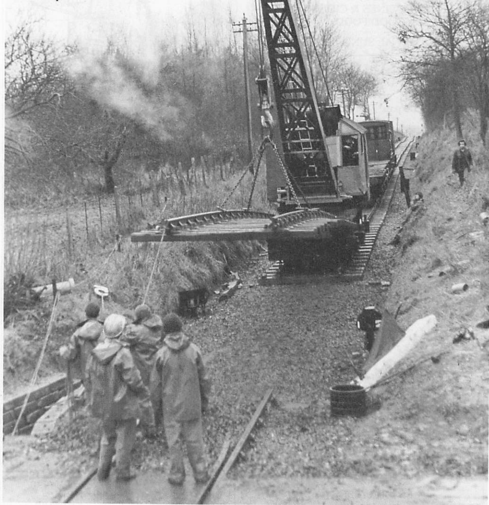
Dropping a wooden sleeper panel into position, 22nd December 1983
