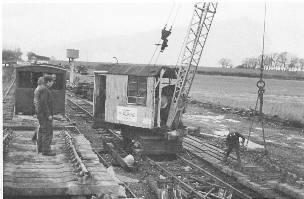
Loading concrete sleepers at Wittersham Road on 2nd January 1984
