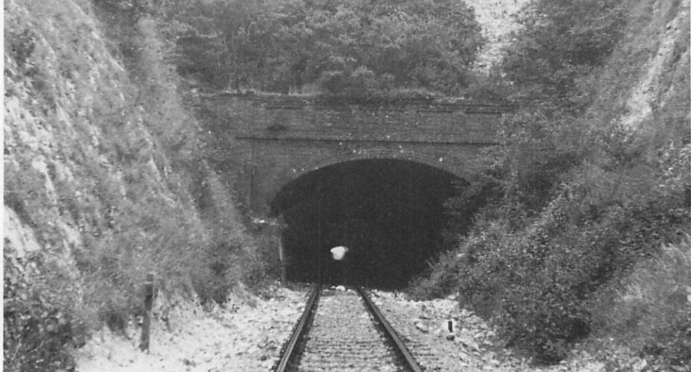
Golgotha tunnel, Shepherdswell end. The gradient post on the left marks the transition from a short stretch of level track to a fall through the tunnel of 1 in 100
