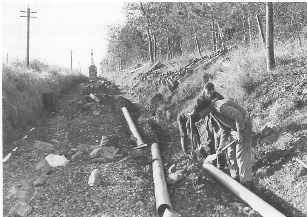
Pitching the new drains, 22nd November 1983
