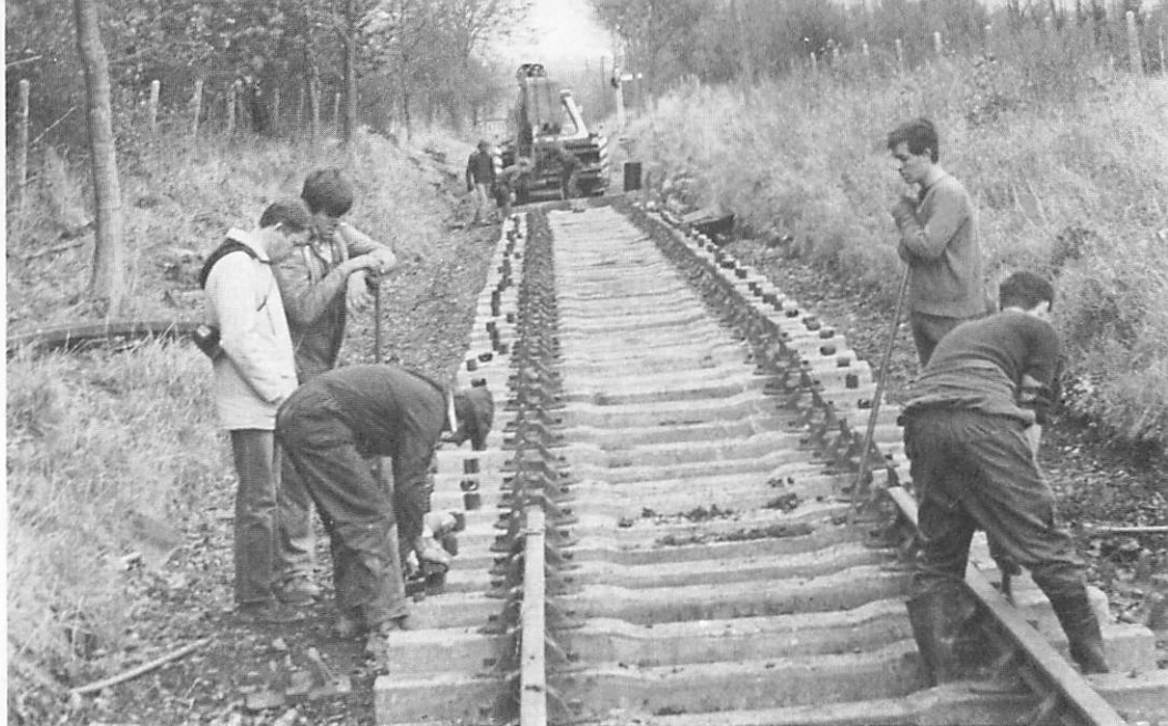
Sleeper relaying near the summit, 30th November 1983
