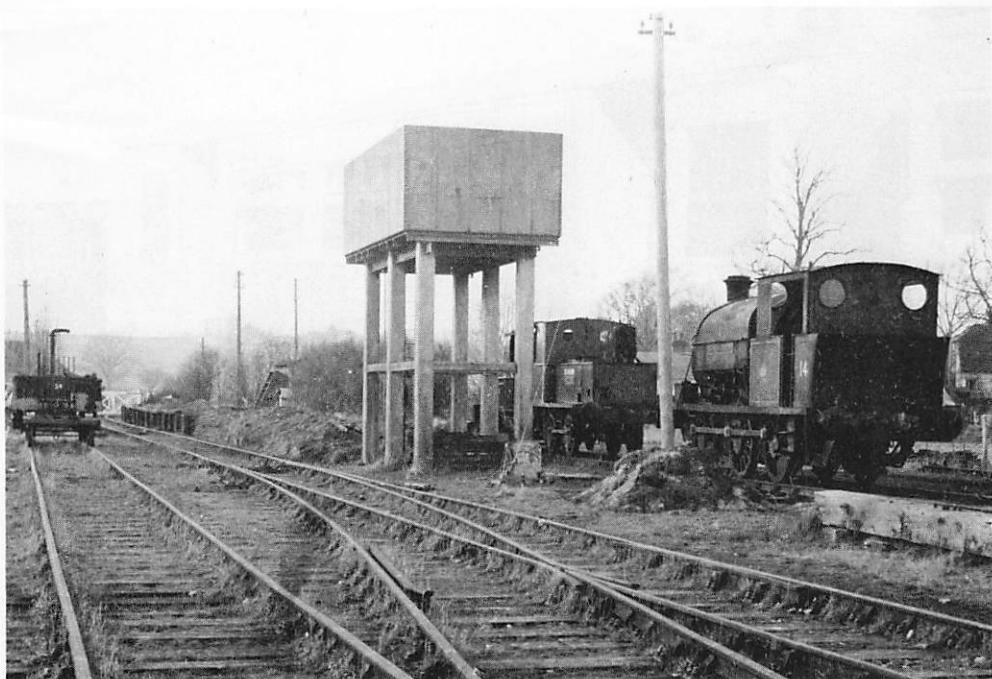
The Rolvenden water tower in the early days of the preservation movement before 'boxing in'. The tank is resting on girders salvaged from No. 6 [S.R. Garrett collection]
