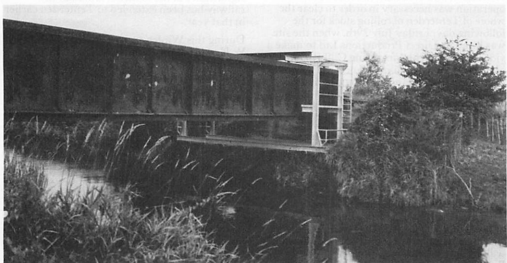
The new travelling platform cradles the Rother Bridge, 17th August 1983.
