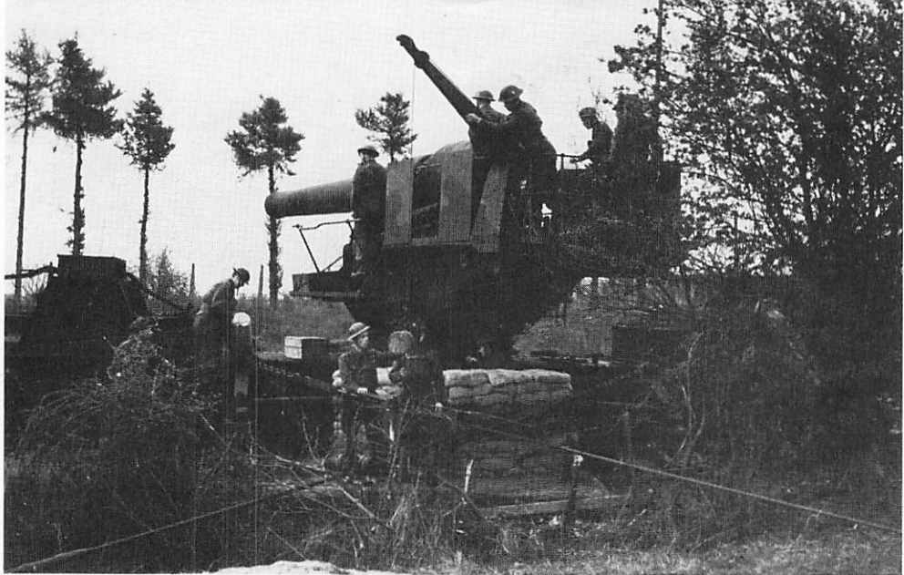
Loading the gun with a 9.2 in shell – note the hoist
