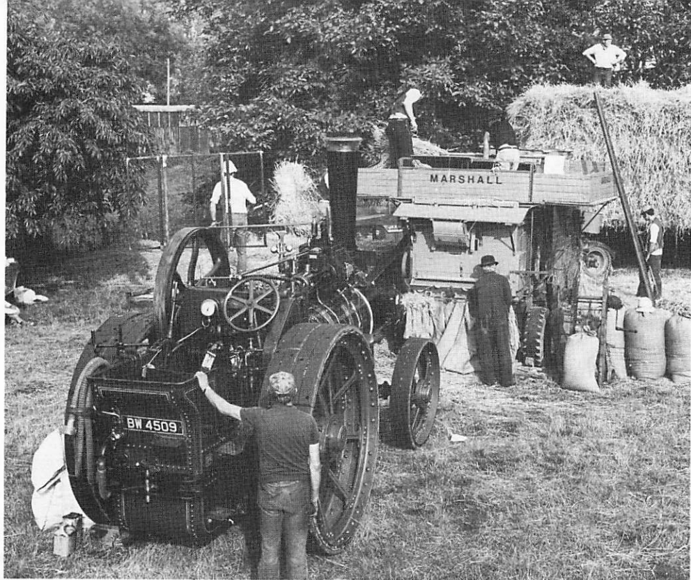
1908 Marshall engine, "Old Nick" driving 54" Marshall threshing drum of 1940 vintage, together with a Massey Harris Trusser of 1930. [Brian Stephenson]
