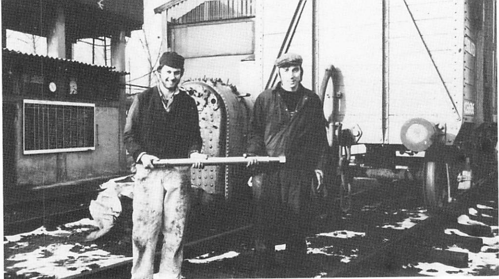
Lawrence Donaldson (left) with one of the two new piston rods he has made for the 'P' class. Paul Norrington supports the other end. (Paul Sutton)
