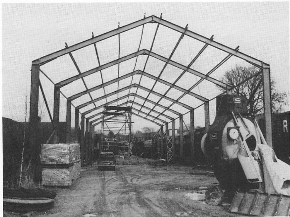
The Carriage & Wagon shed – basic steelwork complete March 14 1981. (Paul Sutton)
