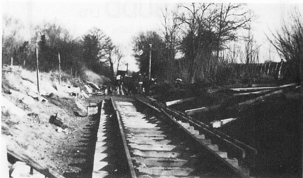
Pre-assembled track panels being laid, February 1980.
