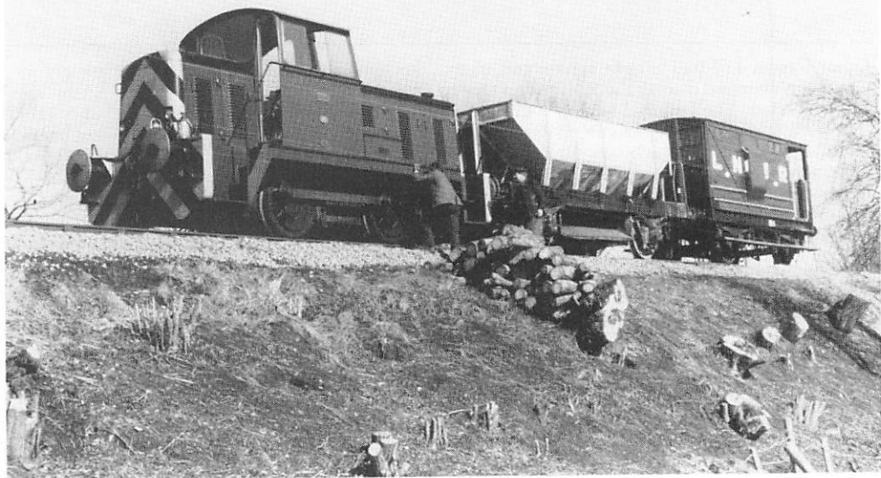
0-4-0D locomotive "Baglan" with a ballast train near Haystacks crossing, February 1978. The ballast has already been laid and the work of the clearance department in the area is also apparent. [John Liddell]
