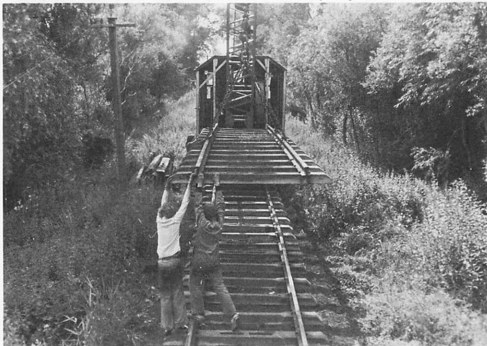
Laying track panels between Wittersham Road and Northiam
