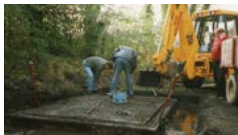
The weighbridge being removed to store.
